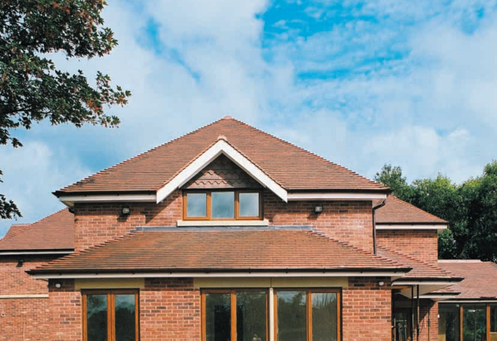
Above: The Brown Brindle Smoothfaced tiles on this private house in Lancashire, complement the lighter multi-coloured brickwork. The use of arris hips provides a neat finish to the hip lines on this stunning property.
