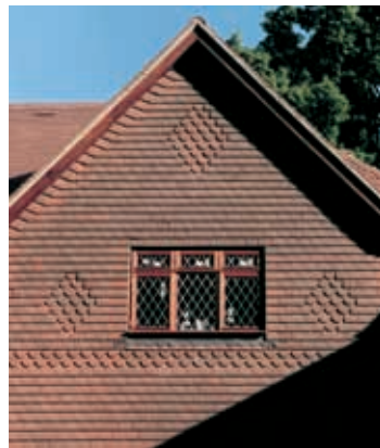
Left: Brown Heather tiles have been used on the roof and vertical tiling on this house. Skillful and imaginative use of ornamental club tiles has enhanced the appearance of this building.
