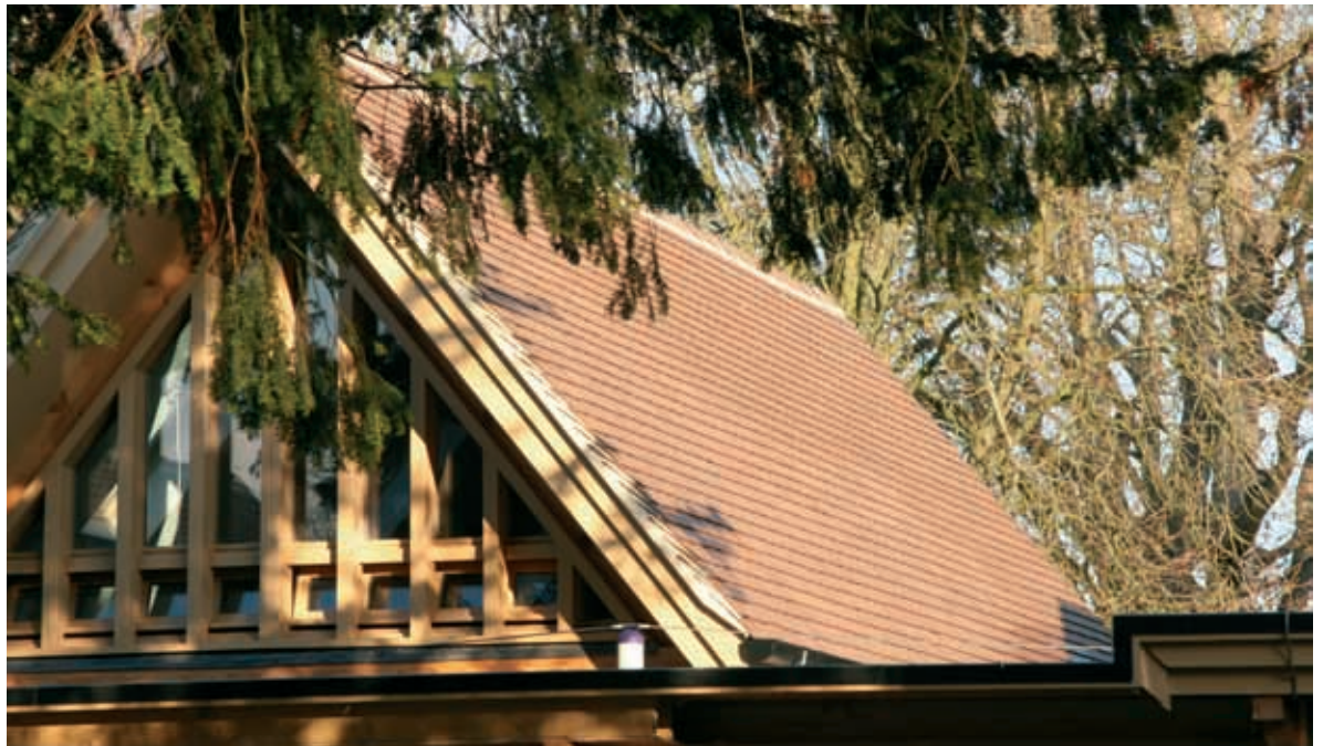
Right: Brown Heather Sandfaced tiles were chosen for the redevelopment of Micheldever Primary School.
