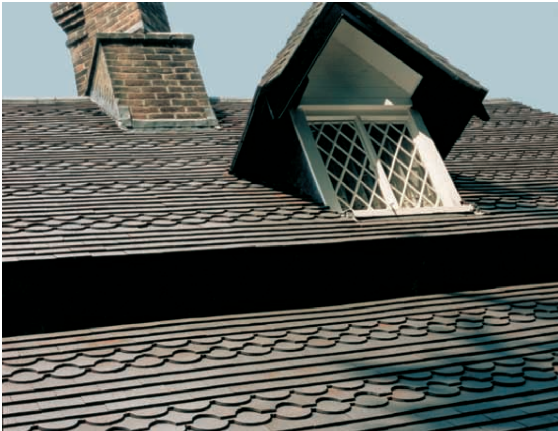
Left: Blue Brindle Tiles have been broken up by the use of ornamental banding used in 3 courses – Club/Fishtail/Club.
