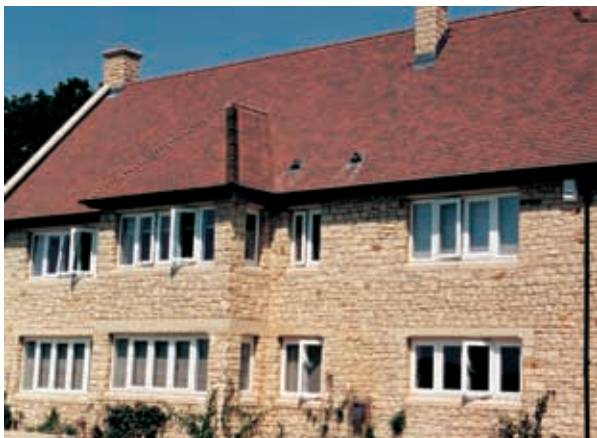
Left: Trafalgar Blend , on a private house near Bridport.
