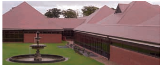
Above: A mixture of Brown Brindle and Brown Antique tiles were used to match up existing tiles no longer in production after a disastrous fire at the National Motorcycle Museum.
