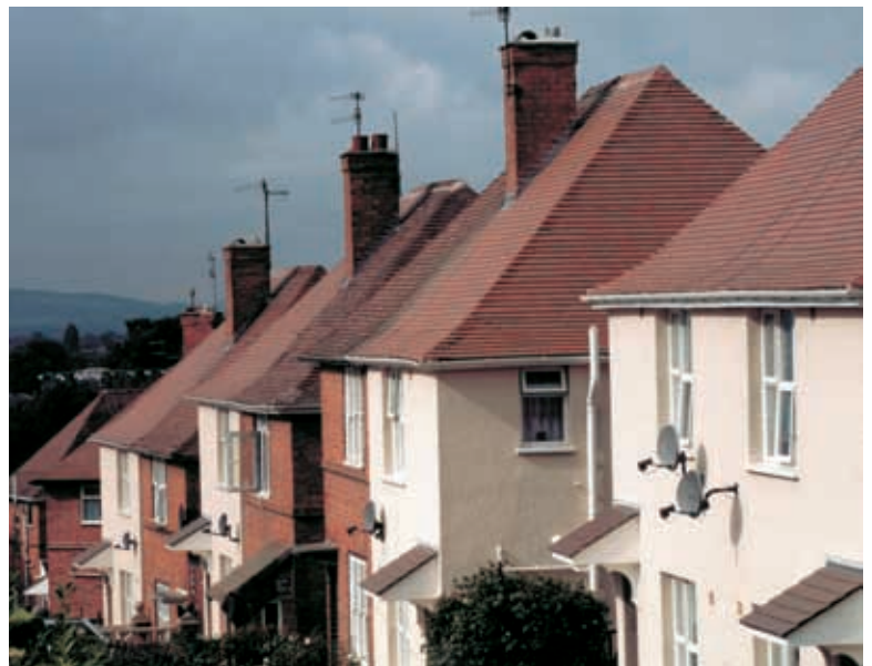
Above: Traditional single camber Country Brown Smoothfaced tiles were used on this re-roofing contract at Tolladine, Worcester.
