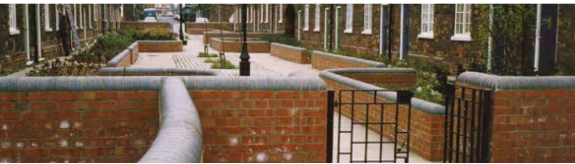
Blue half round cappings at Scunthorpe in a refurbishment scheme for Northern Countries Housing Association. Architects: Michael Hyde & Associates
