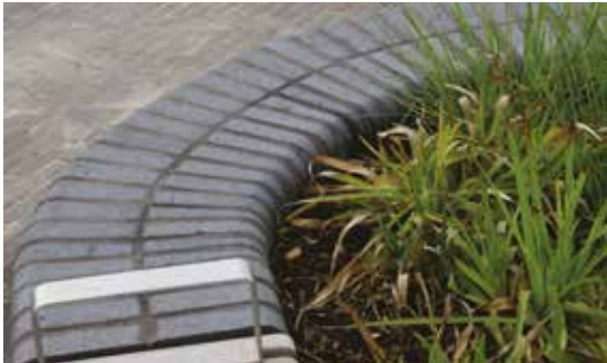
Tapered special bricks in Staffordshire blue at Wichelstowe
