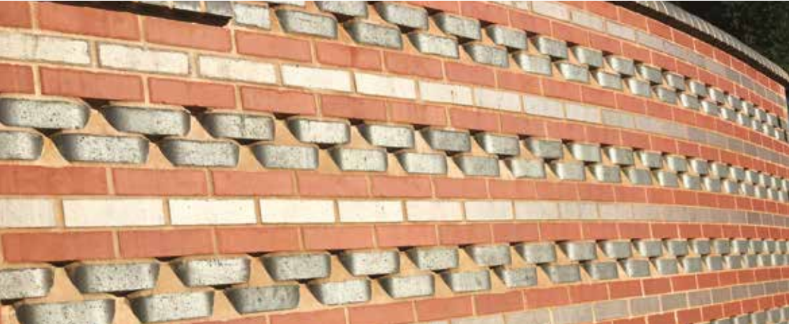
Blue double bullnose bricks create detail on this wall which is capped with blue half round copings.
