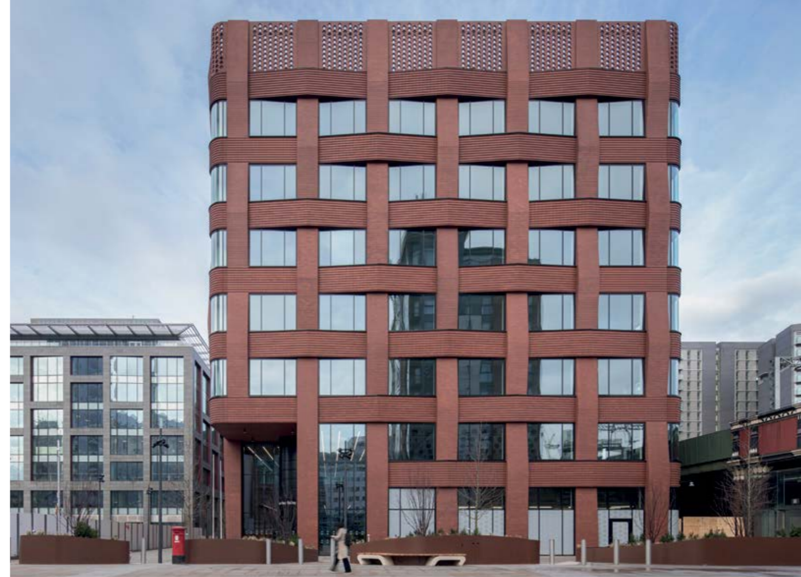
Above: Three New Bailey, the new HMRC building in Salford. This Surface Design Award and Facade Award winner uses Ketley bricks, extruded slips and specials all in Staffs red to create its innovative woven facade.
