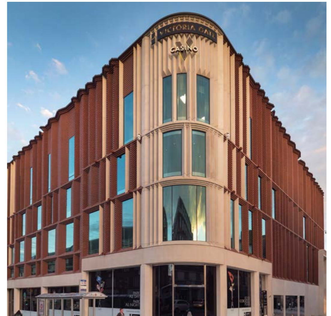
Above: Three New Bailey, the new HMRC building in Salford. This Surface Design Award and Facade Award winner uses Ketley bricks, extruded slips and specials all in Staffs red to create its innovative woven facade.
