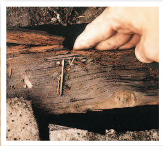
The consequences of inadequate roofspace ventilation
