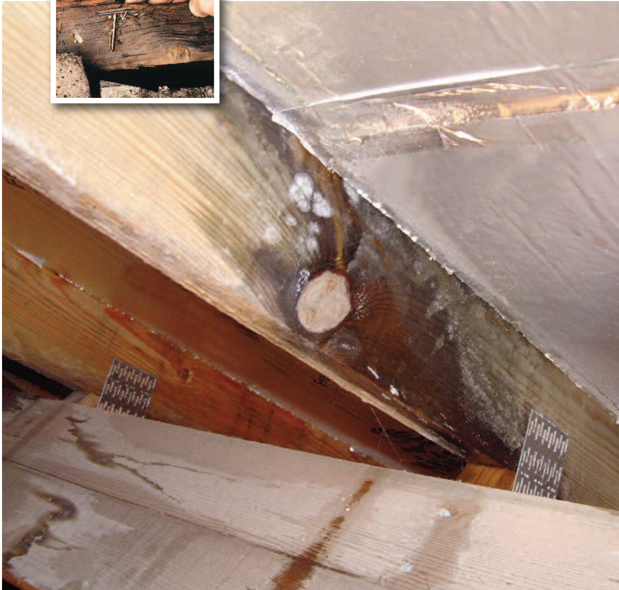
The consequences of inadequate roofspace ventilation
